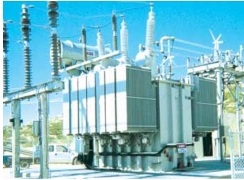
Fig. 1-3 87.5 MVA, 138/34.5 kV Transformer from Hitachi ABB Power Grids [HITACHI ABB POWER GRIDS, 2015]
