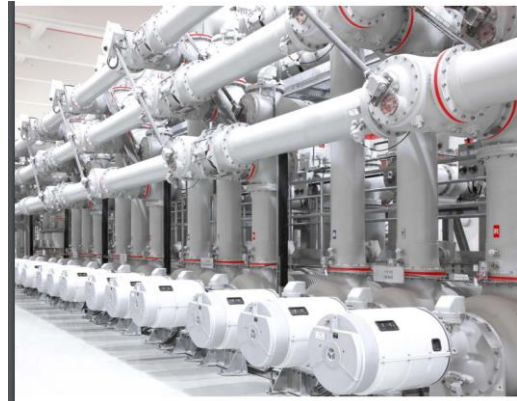
Fig. 1-2 (A) (Left) Gas-insulated switchgear from Hitachi ABB Power Grids (B) (Right) Gas-insulated switchgear ELK-4 up to 800 kV from Hitachi ABB Power Grids [HITACHI ABB POWER GRIDS, 2020a] [HITACHI ABB POWER GRIDS, 2015]
