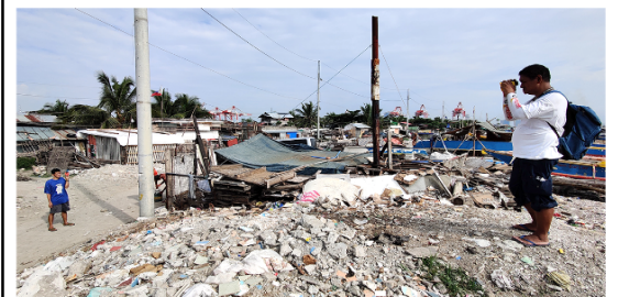
Elevation survey measuring the points D4 and D5. This is an inner rubble mound that residents maintain as part of coastal defense.
