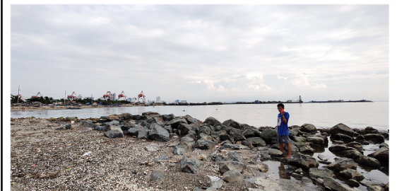
Heavily damaged slope protection created in 2008 near Point C1.
