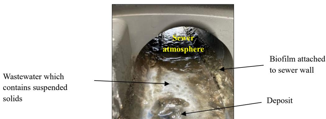
Figure 1. A sewer where the microbial activity and chemical reaction occur
