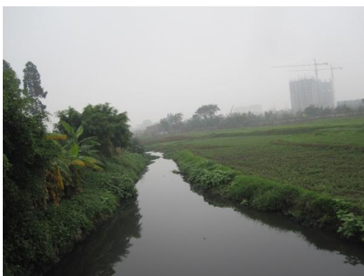
Figure 12. Drainage canal in Thanh Liet
