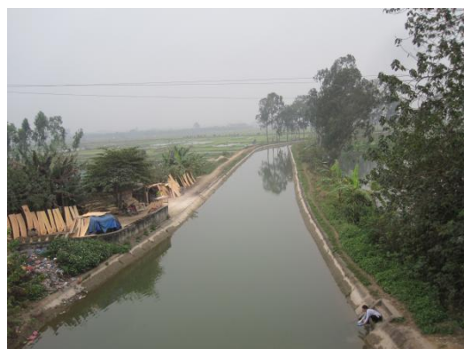
Figure 15. Irrigation channel from Dan Hoi water gate
