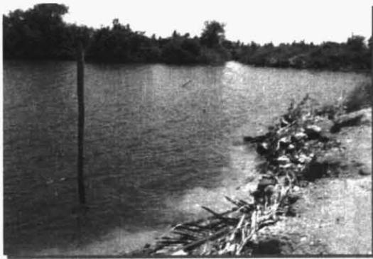
Degraded Water at Closure Dam
