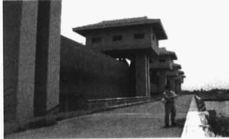
Diversion Dam, a close look (1)
