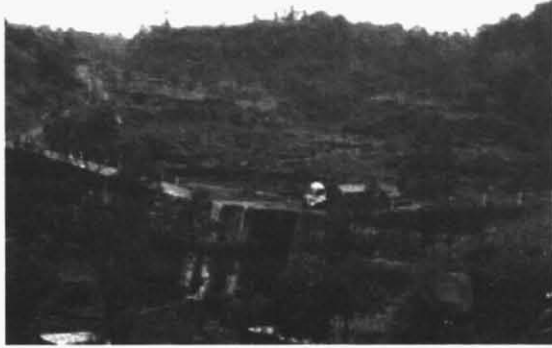
Dam on the Apu River, Merapi (JBIC, 2003)
