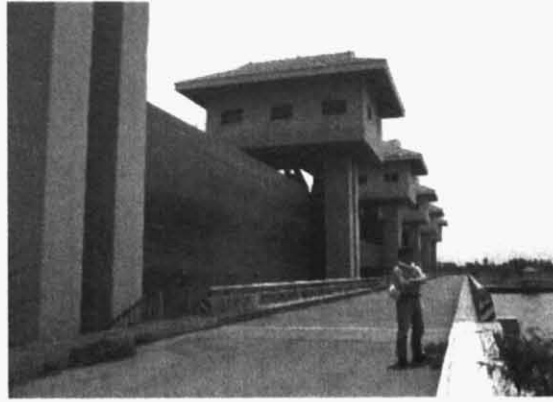
Diversion Dam, a close look
