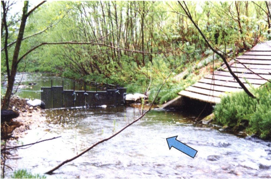
Fig. 5.2a A partial fence installed above the Soya Research Branch of the Hokkaido Fish Hatchery. The allow indicates flow direction.
