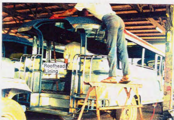
Installation of roofhead lining.
