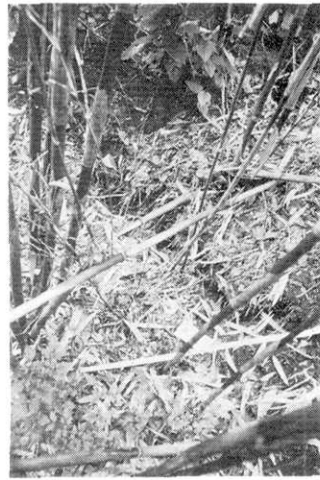
Fig. 31. Crack at Loc. 27, the northern end of the Irozaki-median Fault.
