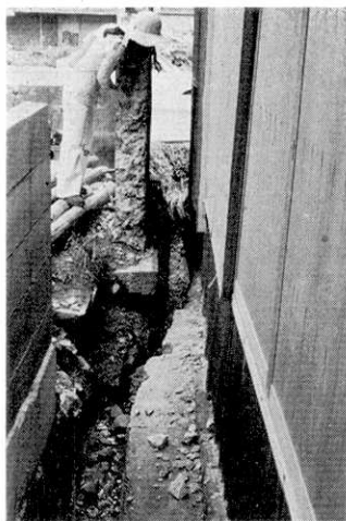
Fig. 16. Offset of ditch at Loc. 9.
