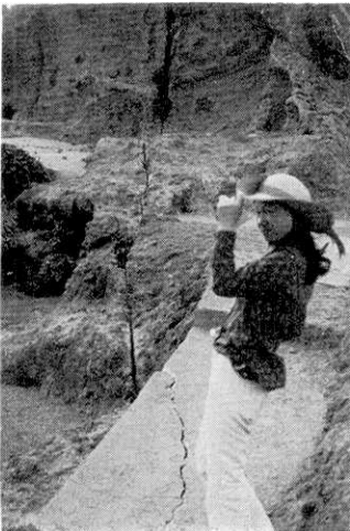
Fig. 42. Crack at Irozaki Point.
