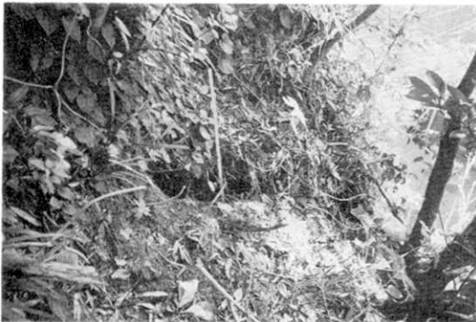
Fig. 12. Crack on slope near Loc. 5.
