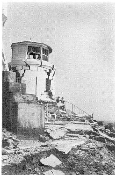
Fig. 7. Destruction of a building made of stone blocks at Irozaki.
