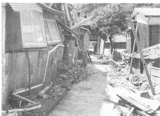
Fig. 5. The damage at Iruma.
