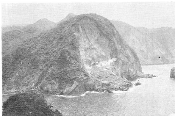
Fig. 11. Rock fall along the coast at Iruma.
