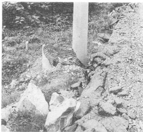
Fig. 65. Destruction of a pole at loc. G-20.
