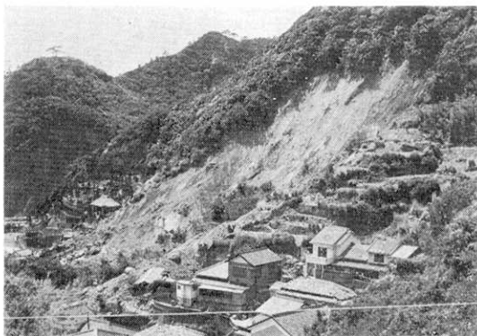
Fig. 9. Landslide at Nakagi.
