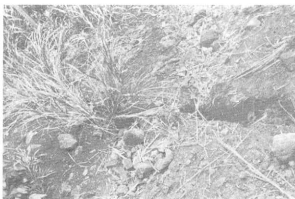
Fig. 67. A fissure in the ground at loc. G-21. (By Dr. M. HAKUNO.)
