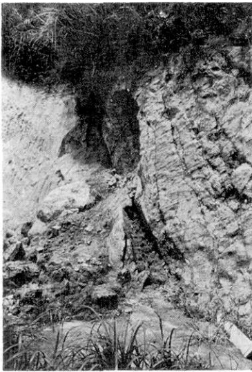
Fig. 80. Earthquake fault at loc. R-13.
