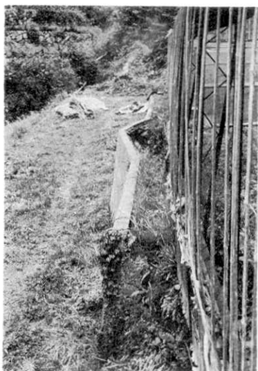
Fig. 85. A fissure in the ground at loc. G-30.
