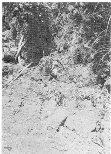
Fig. 50. Fissures in the ground at loc. G-9.
