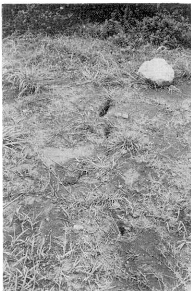
Fig. 70. Fissures in the ground at loc. G-25.
