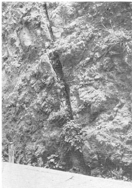
Fig. 62. Earthquake fault at loc. R-10.
