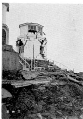
Fig. 35. Damage to a stone masonry observation platform at Irozaki.
