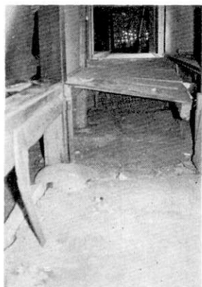
Fig. 29. Movement of columns from independent footings at Iruma.
