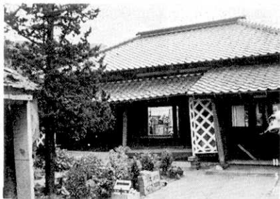
Fig. 25. Damage to a house at Iruma. Roof tiles did not suffer damage.
