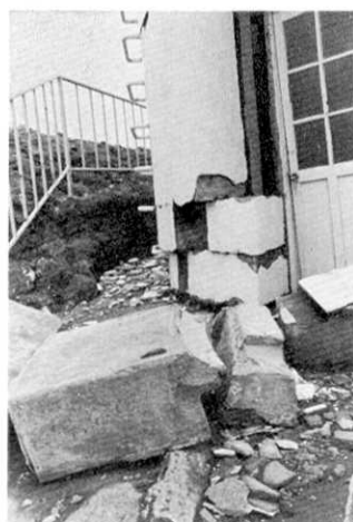
Fig. 36. Detail of a damaged stone masonry observation platform at Irozaki. The size of a stone is indicated by a comparison of it with a shorehorn.
