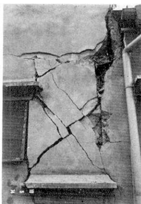
Fig. 14. Detail of damaged reinforced concrete building at Nakagi.
