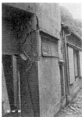
Fig. 13. Damage to a reinforced concrete building at Nakagi.
