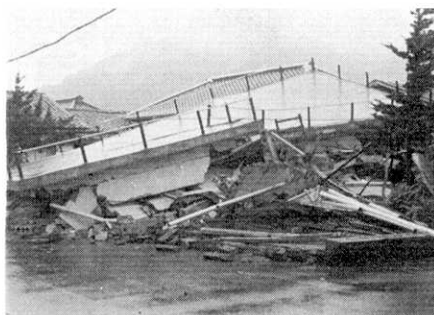
Fig. 16. Complete collapse of a concrete block masonry building at Iruma.
