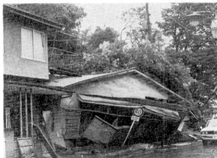
Fig. 39. Damage to a house caused by falling rocks at Shimokamo.
