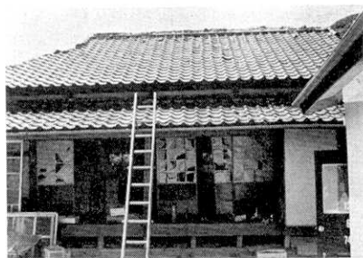
Fig. 20. Damage of a house. Roof tiles suffered damage. (at Iruma)
