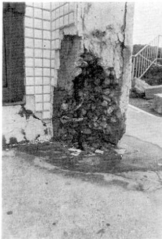
Fig. 38. Detail of a damage to a reinforced concrete tower at Irozaki.
