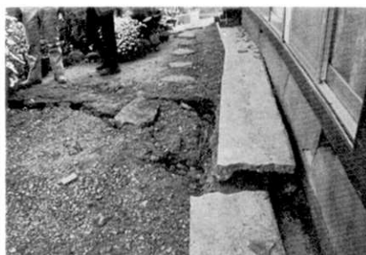
Fig. 34. Damage to a house on a fault at Irozaki.
