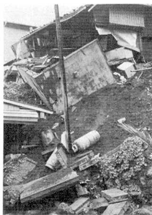
Fig. 18. Destruction of a fence and a house caused by ground failure at Iruma.
