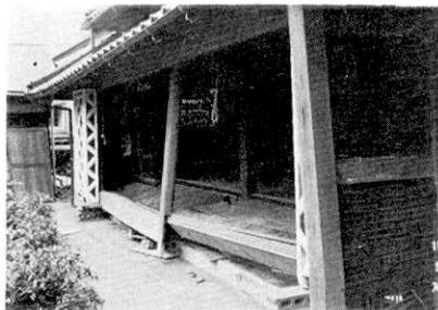
Fig. 26. Detail of a damage of sill at Iruma.
