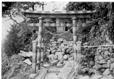
Fig. 56. Destruction of stone pitching at Ochii.
