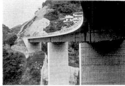
Fig. 19. Isuzu girder bridge.
