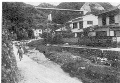
Fig. 12. Tengu truss bridge.
