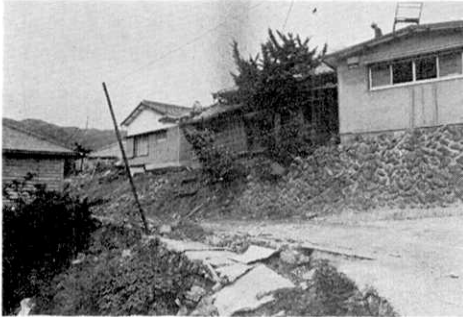
Fig. 35. Fault passage through a thick sand deposit.
