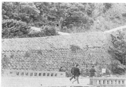
Fig. 6. Swelling of stone pitching.
