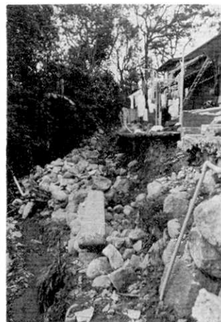
Fig. 55. Sliding of the supporting soil of a house garden at Ochii.
