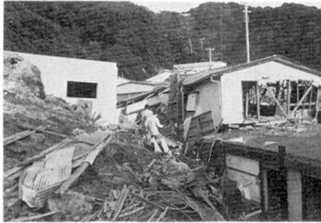
Fig. 46. Houses destroyed by the landslide.
