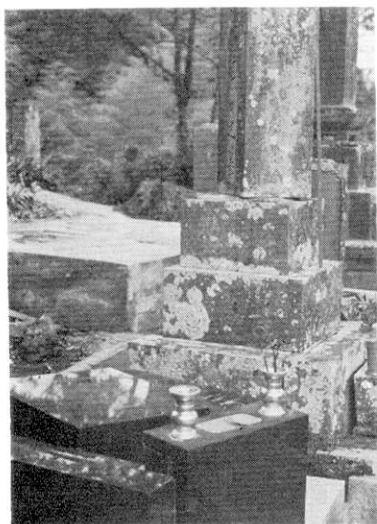
Fig. 9. Rotation (angle 137^\circ ) and overturning of gravestones at Shimo-ono.
