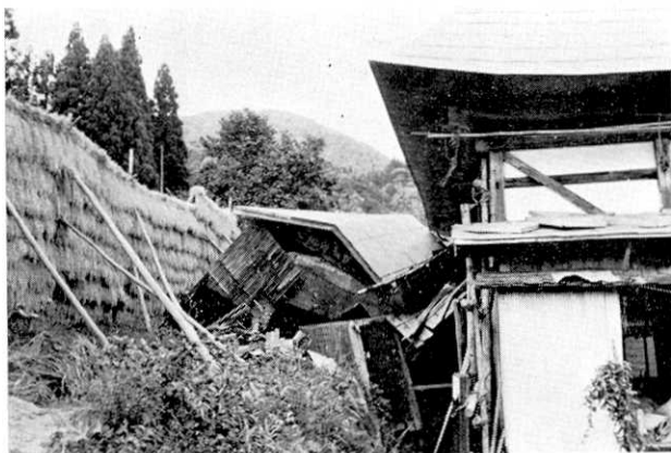
Fig. 11. Collapse of a detached room at Iwaigawa, Higashinaruse-mura.
