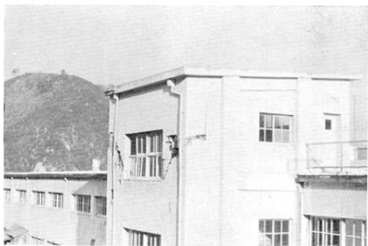
Fig. 21. Failure of the concrete-block wall of Kawajiri Elementary School, Yuta-machi.
