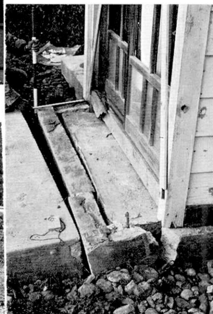
Fig. 20. Sift of a house from its concrete-base at Mitsumata, Sennaimura.
