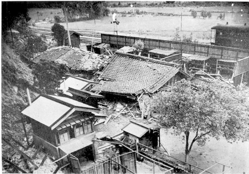
第 164 圖 内埔庄. 大安驛官舎 (木造) の倒潰. Fig. 164. Naiho-syô, Taian railway station. Collapse of the residence (wooden structure) of the station master.
