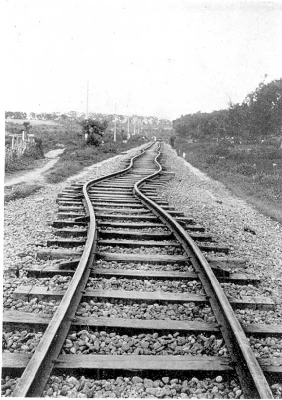
第 173 圖 内埔庄后里驛北方約 700 m に於ける軌條の波狀屈曲. Fig. 173. The sinuous bucklings of rails, 700 m north of Kōri station, Naiho-syō.
