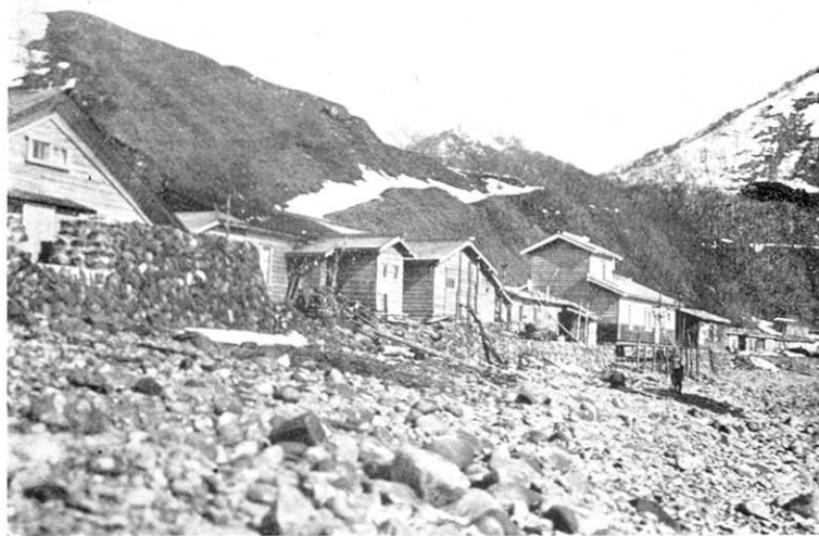
第 219 圖 庶野の海岸. 左端の防浪堤は津浪に對しては有效であつた. (4 月 6 日那須撮影) Fig. 219. Seashore of Syoya. The breakwater seen at l. h. side of photo saved the house from the tsunami. (Photo by N. Nasu, April 6.)
