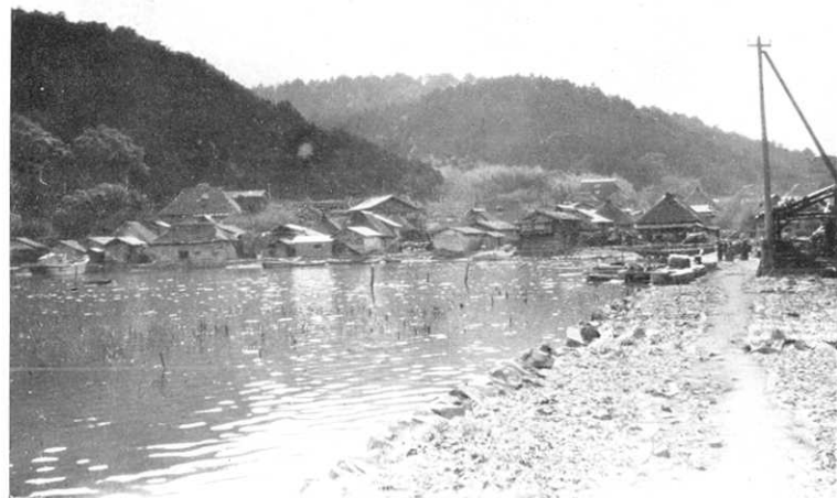
第 402 圖 大原村小淵。写真は小淵の細長き入江の最奥の部分を示す。家は皆床上3~4尺は浸水したるも倒壊せず。写真右端の家にて浪高平均海面上2.9米。(5月23日高橋撮影) Fig. 402. Kobuti, Ohara-muru. The water reached the floors of the houses shown in the photo, but did not demolish them. The height of the tsunami was 2.9 m above sea level on the wall of the house under the arrows. (Photo by R. Takahasi, May 23.)
