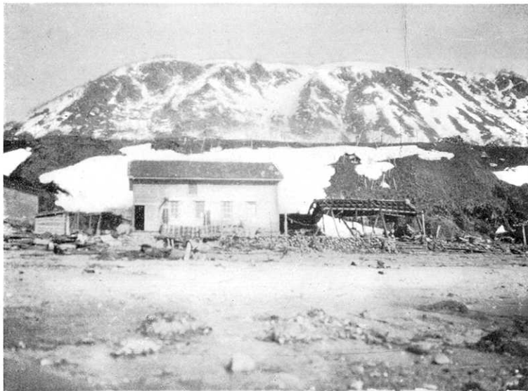
第 217 圖 庶野東端に於ける家屋被害。(4月6日那須撮影) Fig. 217. Damaged houses in the eastern part of Syoya. Weatherboards of the house (middle) were ripped off by the tsunami. (Photo by N. Nasu, April 6.)
