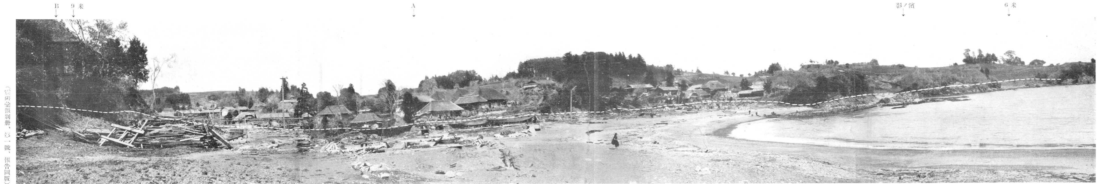
第 335 圖 小友村唯田。圖中點線では津浪の最高點の跡を示めてゐる。圖上に矢をもつてその附近での浪高を示してある。A 附近で流された家は皆影ノ濱に流され岸にあがつてゐた。B 附近は長洞部落に屬した所であるがこの所は 9 米、影ノ濱附近では 6 米と浪高はなつてゐる。唯田では流失 7 軒、半壊 1 軒を出し、4 人流死してゐる。(4 月 30 日西村、高山撮影) Fig. 335. Tadaide, Kotomo village. Dotted line shows maximum heights reached by tsunami; the same for particular points being indicated by arrows. All the houses that stood near "A" were found washed up on Kagehama beach, where wave height was 6 m. In the neighbourhood of "B" (Nagahora hamlet) wave height was 9 m. At Tadaide, 7 houses with 4 persons were washed away and 1 house partly demolished. (Photo by G. Nishimura and T. Takayama, April 30.)
