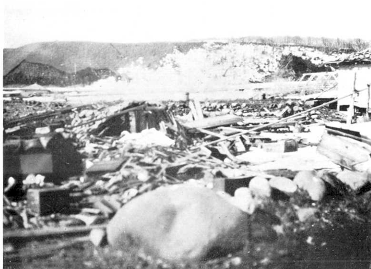
第 220 圖 鹿野シトマン川河口に於ける倒壊家屋。(4月6日那須撮影) Fig. 220. Houses at the mouth of the Sitoman River demolished by tunami. (Photo by N. Nasu, April 6.)
