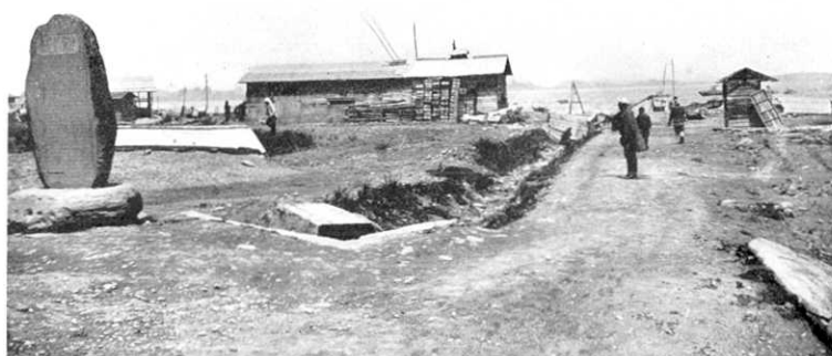
第 361 圖 大谷村大谷. 津浪前は此の邊一帶に住宅及納屋ありしも皆流失す. 津浪は寫眞左手の明治 29 年の海嘯記念碑の頂下 5 寸程迄届きたりと云ふ. 此の邊津浪の高さ平均海面上 4.5 米. (5 月 18 日 高橋撮影) Fig. 361. Oya, Oya-mura The houses & cottages which stood before the tsunami were all washed away. The water reached a height of 15 cm beneath the top of the stone-monument (the monument of the tsunami of 1896) shown at the left of the photo. (Photo by R. Takahasi, May 18.)
