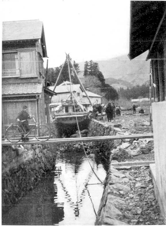
第 404 圖 女川町魚市場附近。道路を越して堀割に 嵌入せる漁船。(3月4日高橋撮影) Fig. 404. Onagawa-mati. A large fishing boat driven right into a ditch, cutting one of the main roads. (Photo by R. Takahasi, March 4.)
