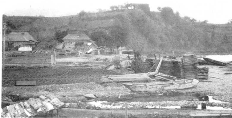
第 382 圖 戸倉村長清水. 海岸の納屋及住宅流失す. 浪は寫眞の矢印の家の右側に地上 1 尺程浸水せり. 浪高 4.5 米. (5 月 21 日 高橋撮影) Fig. 382. Nagasuzu, Tokura-mura. The water reached the foundation of the house shown under the arrows. (4.5 m above sea level.) Cottages situated at lower levels were washed away. (Photo by R. Takahasi, May 21.)
