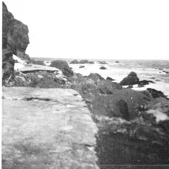
第 213 圖 サクバイ附近道路の破壊。(4 月 6 日那須撮影) Fig. 213. Concrete road partially destroyed by tsunami near Sakubai. (Photo by N. Nasu, April 6.)
