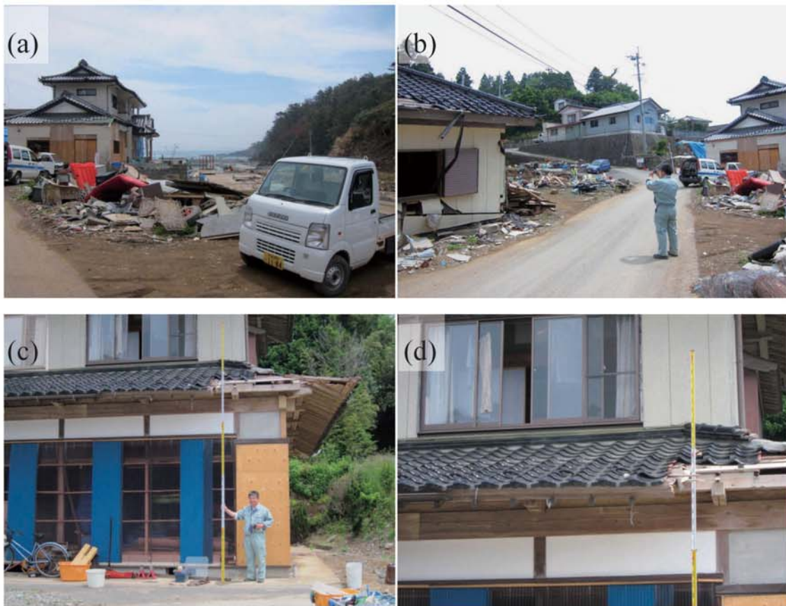
Fig. A160. (a)-(b) Damage at Utatsu-Ishihama. (c)-(d) Tsunami trace survey point on the the roof of Mr. Abe's house (4.10 m above ground level, M25).
