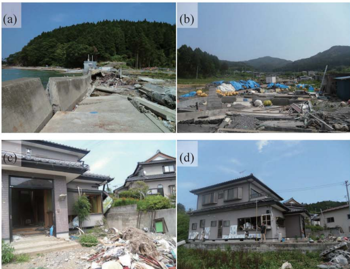
Fig. A176. (a)-(c) Damage at Takihaman. (d) Tsunami trace survey point on the roof of a house (2.75 m above ground level, M36).
