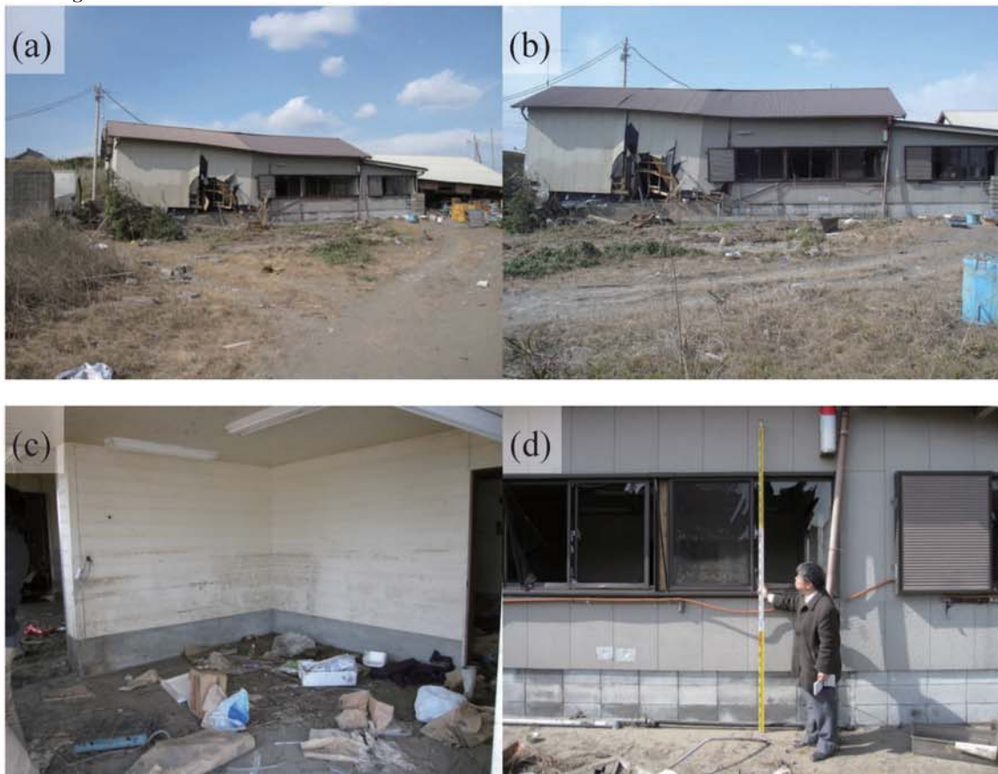
Fig. A302. (a)-(b) The building of a marine product-processing factory destroyed by the tsunami. (c)-(d) Watermark on a wall of a marine product-processing factory (1.94 m above ground level; C7).
