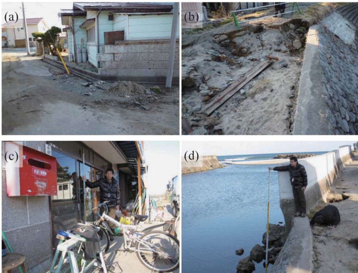
Fig. A252. (a)-(b) Damage at the side of the Sekine River in Hizenzo. (c) Watermark on windowpanes of entrance sliding doors of the sign factory Kibokogei at the riverside in Hizenzo (0.73 m above ground level, B11). (d) Measuring ground height at the survey point based on the water surface in the Sekine River.
