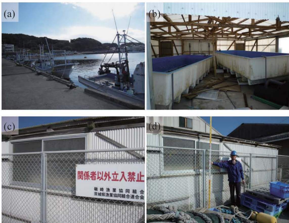
Fig. A278. (a) Isozaki Fishing Port. (b) Damage to shed in Isozaki Fishing Port. (c)-(d) Watermark on windowpanes of shed at the port (1.76 m above ground level, B27).
