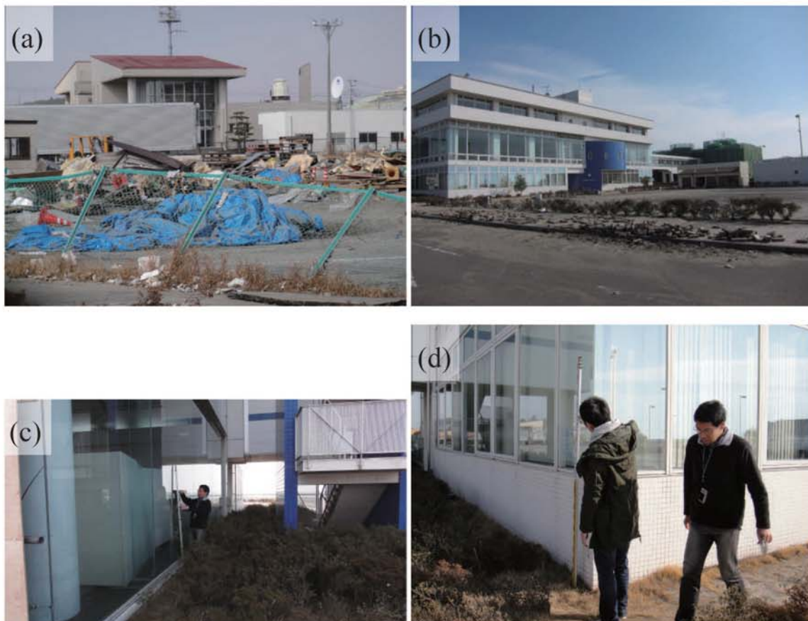
Fig. A284. (a) Damage at Minatochuo (Ibaraki Port, Oarai District). (b) Ferry terminal building at Oarai Port. (c) Watermark on windowpanes of ferry terminal building (1.575 m above ground level, B30). (d) Another watermark on windowpanes of the ferry terminal building (1.65 m above ground level, B31).
