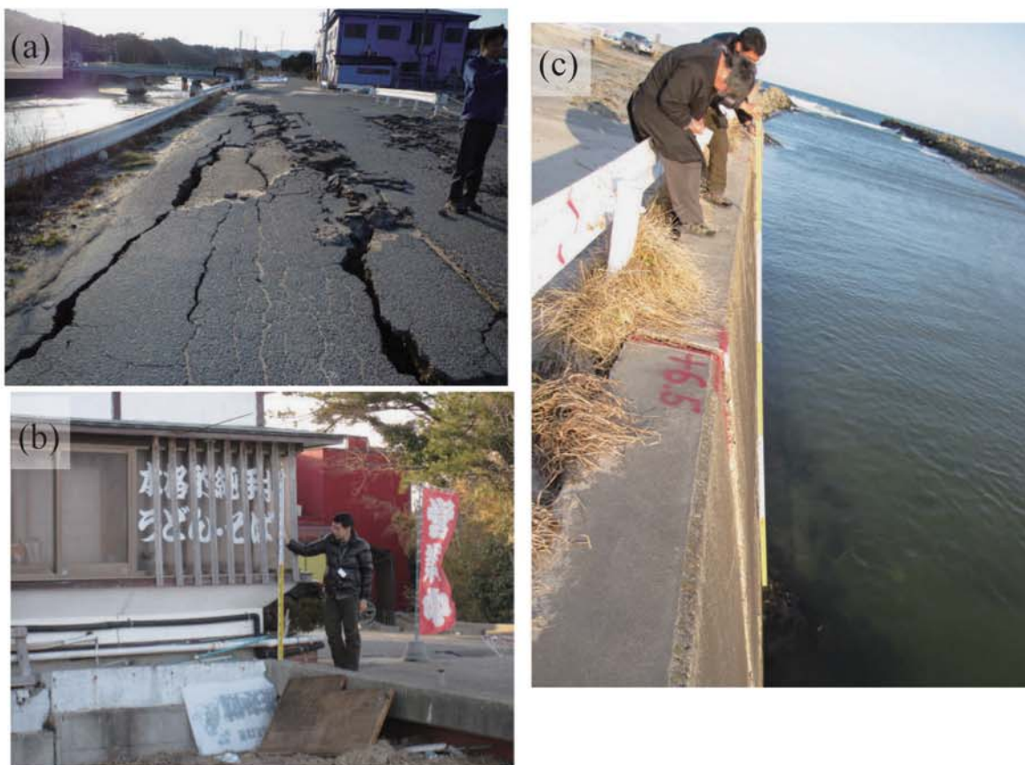
Fig. A254. (a) Liquefaction along the Hananuki River in Arakawa. (b) Tsunami trace survey point at the parking lot of the restaurant Sanukijaya (B12). Tsunami inundated the top of the slope at the parking lot. (c) Measuring ground height at the survey point based on the water surface in the Hananuki River.
