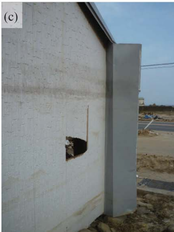
Fig. A248. (a)-(b) Damage at Isoharacho-Isohara. (c) Watermark on the wall of the building of the Murata Ironworks. (d) Tsunami trace survey point at the Murata Ironworks (2.03 m above ground level, B9).
