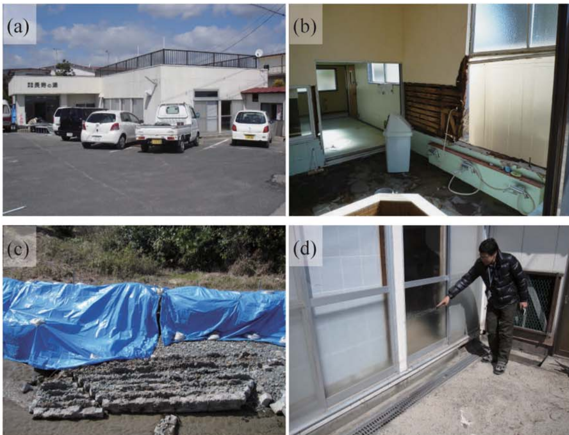
Fig. A262. (a) The spa Chojunoyu at the side of the Kita River in Higashinamekawacho (tsunami trace survey point). (b) Damage at the bathroom of the spa Chojunoyu. (c) Damage to riverside walls caused by the tsunami flowing backward in the Kita River (testimony of spa staff). (d) Watermark on windowpanes of the spa Chojunoyu (0.89 m above ground level, B17).
