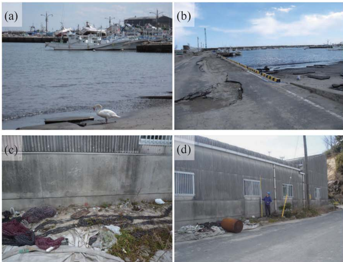
Fig. A272. (a)-(b) Damage at Kuji Fishing Port. (c) Debris and fishing nets on the road beside a warehouse in the port. (d) Tsunami inundation limit based on scattered debris (under the rod, B24).
