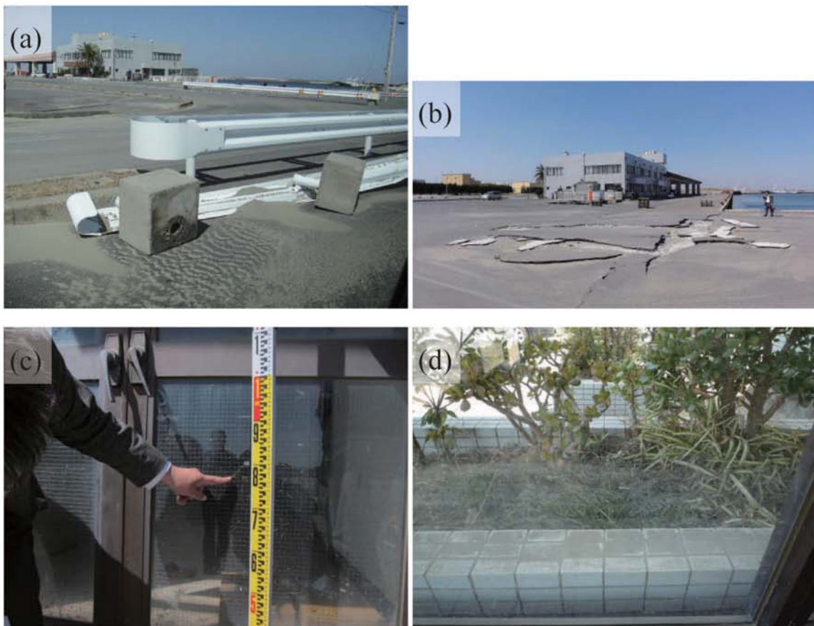
Fig. A290. (a)-(b) Damage around the fishery association building in Shin Fishing Port. (c) Watermark on the entrance doors of the fishery association building (0.898m above ground level; B36). (d) Watermark on a windowpane of the fishery association building.
