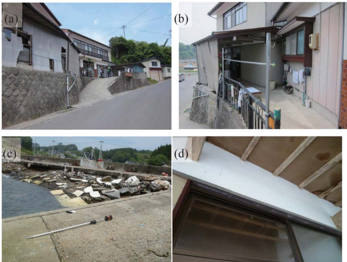
Fig. A166. (a)-(c) Damage at Utatsu-Nirano-hama. (d) Tsunami trace survey point on a wall of Mr. Abe's house (2.68 m above the dirt floor, M28).
