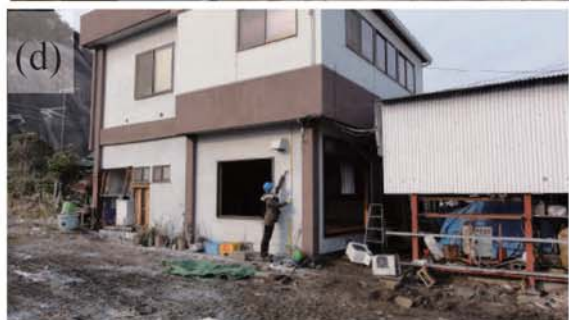
Fig. A248. (a)-(b) Damage at Isoharacho-Isohara. (c) Watermark on the wall of the building of the Murata Ironworks. (d) Tsunami trace survey point at the Murata Ironworks (2.03 m above ground level, B9).
