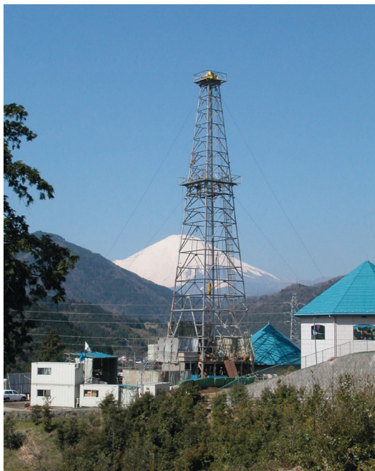
Fig. 2. Photograph of borehole drilling at Yamakita-Minami.
