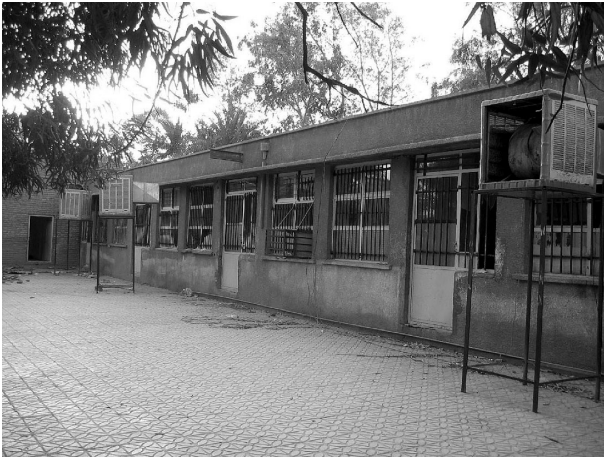
Photo 5. Single-story school building (slight damage).
