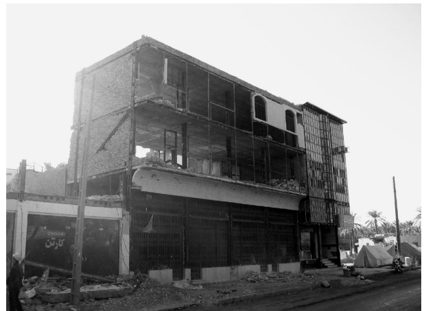
Photo 7. Residence and store building under construction.
