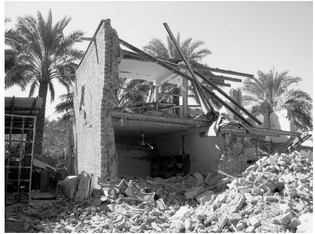
Photo 6. Collapsed two-story school building.
