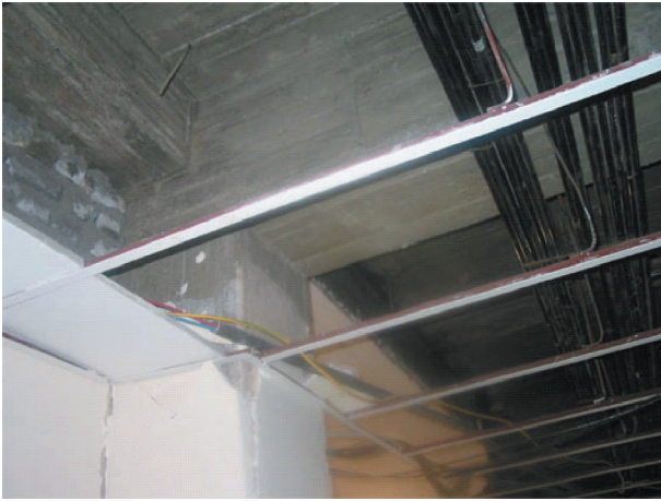
Fig. 21. A beam-column connection on the first floor of the Bam telephone center, which had no damage (about 1,000 m north of the strong motion station).
