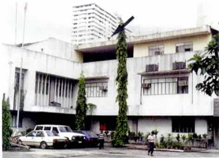
Photo 3. GPS antenna site at Manila. The antenna is set on the roof as shown by arrow.
