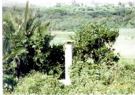
Photo 2. GPS antenna at the Ishigaki site.
