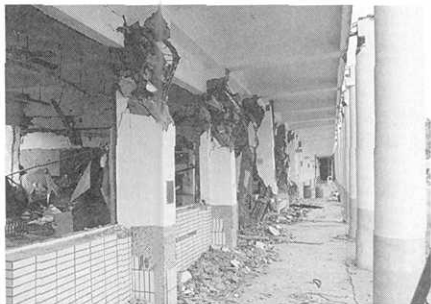
Photo 17. Severely damaged first story of building B at Chungliao National Elementary School
