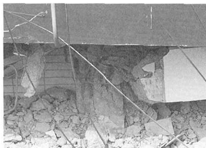
Photo 16. Close-up of Photo 15 (Longitudinal bars buckled although there were many longitudinal bars.)
