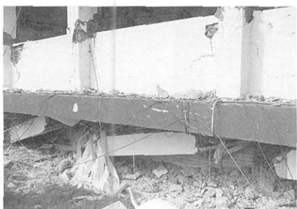
Photo 15. Collapsed first story of building A at Chungliao National Elementary School
