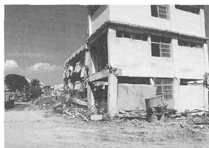
Photo 6. Building A of Nankuang National Elementary School in Puli, which was severely damaged and was being demolished
