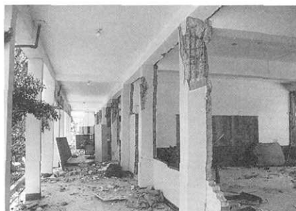
Photo 2. Severely damaged tops of columns at building C of Shikang National Elementary School
