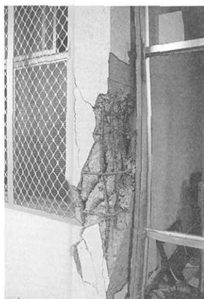
Photo 13. A damaged column by the first story front entrance at Jryetan Meteorological Agency
