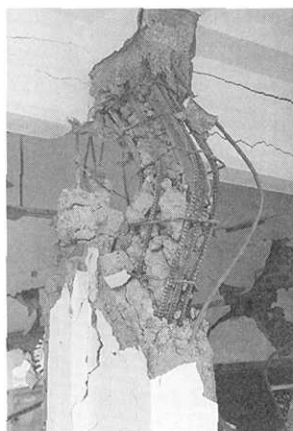
Photo 18. Close-up of Photo 17 (Longitudinal bars buckled. Pipes were found.)
