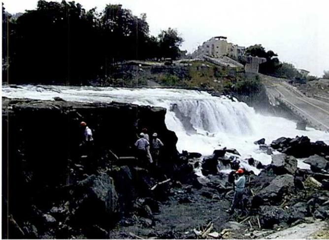
Photo 3. Fall made of the surface fault in the Ta-Chia River (See Fig. 5 for location). The fault is striking NE, and the vertical offset is around 6 m (Otsuki and Yang, 1999). The buildings on the hanging wall had no damage.
