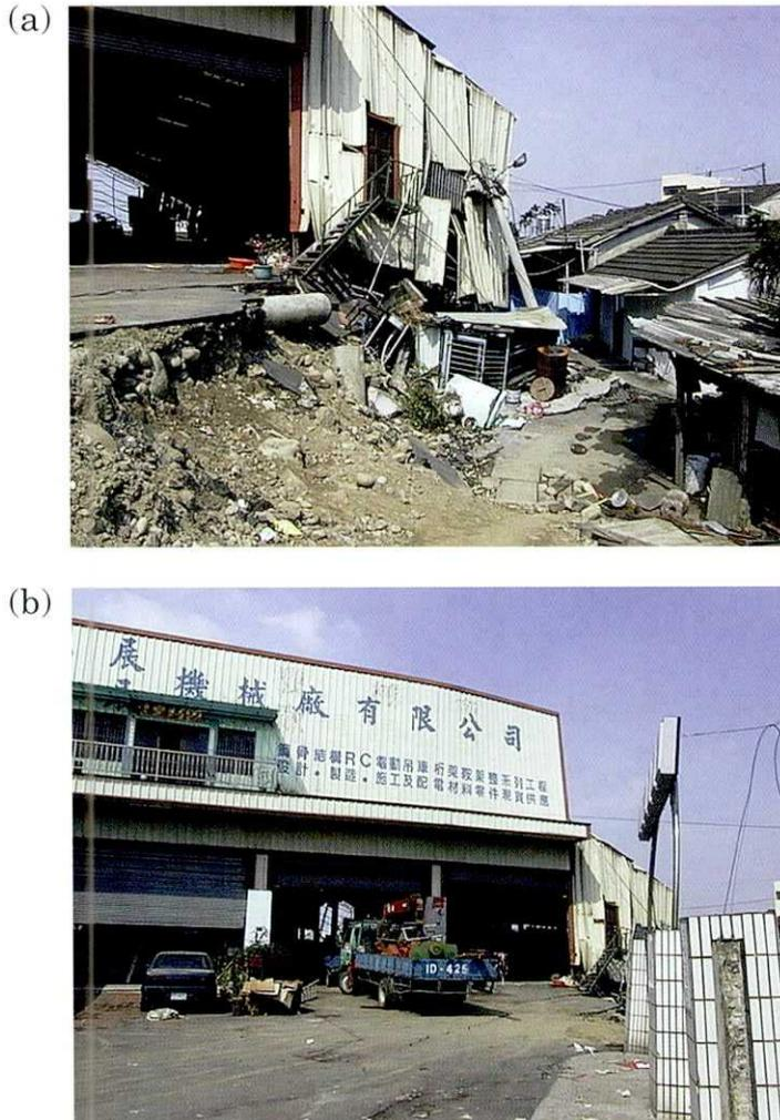
Photo 1. Factory in Chu-Tzu Keng (See Fig. 3 for location). (a) The right side of the factory was severely damaged and was standing over the surface fault, extending NE. (b) On the hanging wall, in the rest of the factory, no damage was seen and the machines were running. The window glass was not broken.
