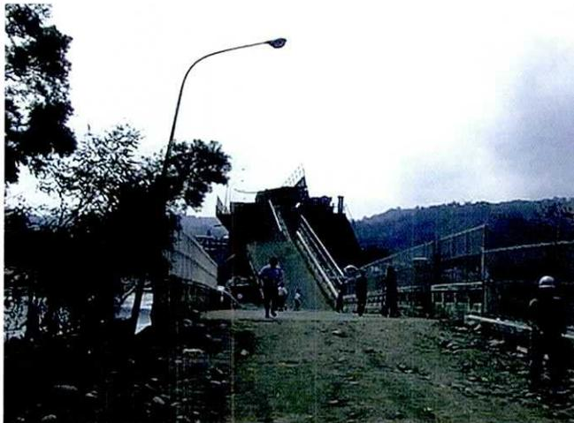
Photo 6. Dam destruction looked from the north (See Fig. 5 for location). The vertical offset is around 9 m (Otsuki and Yang, 1999).
