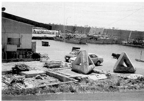
Photo 7. Carried concrete blocks by the tsunami in Kamiura Port in Taisei Town.
