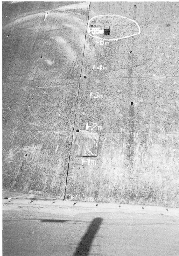
Photo. 5 A "Tsunami-dome-ishi" stone was set before the construction of road at the marked surface of the concrete wall, whose height is 5.5 m from the ground here, and is 9.6 m in TP standard. At Kyodomari, Yokoshima Town.
