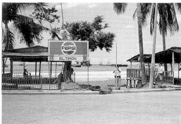
Photo. 11. Sea water rose up to the lower side of the Pepsi signboard (3.6 m) at San Juan del Sur (J in Fig. 34).
