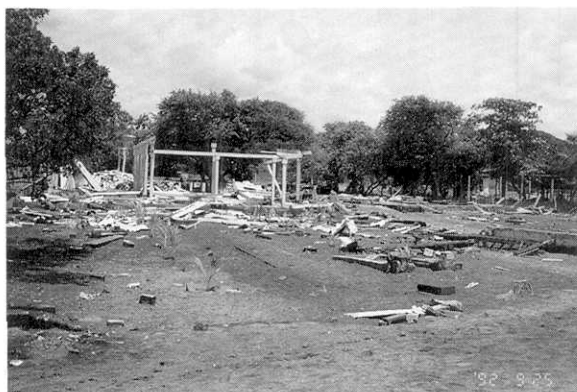
Photo. 5. About 200 houses were entirely destroyed or swept in the residential area of El Transito.
