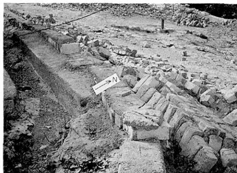
Photo 22. Collapse of a block wall in Pakdeh (Site No. 5 in Fig. 8).
