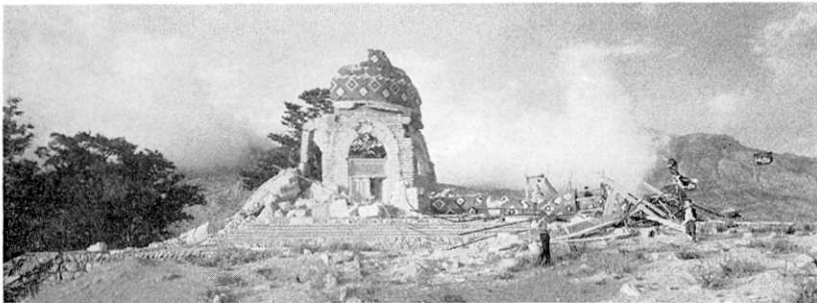
Photo 8. Mosque in Bivarzin. Reinforced brick tower fell down to the ground.
