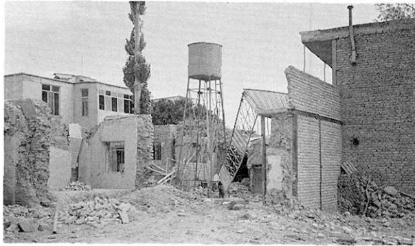
Photo 10. Destroyed adobe houses and an undamaged water tank in Beg Kandi located in the vicinity of Abtorsh, 50 km south of the source area. The death rate was 0.02-0.04% for the 1,600 inhabitants.
