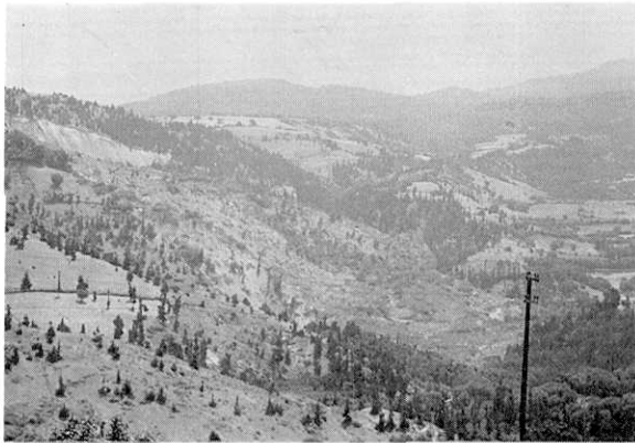
Photo 25. Landslide at Jubon or Ganjeh looking east (Site No. 4 in Fig. 6). A fresh scarp at the left top is the sliding surface. The head of the slump block and debris tearing many trees are seen.
