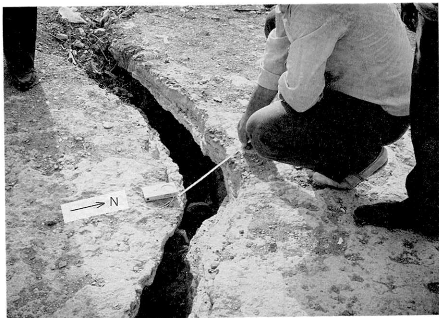
Photo 32. The measurement of cracks on the ground of the calcareous tuff (Site No. 4 in Fig. 8). The horizontal offset was less than 20 cm left laterally.
