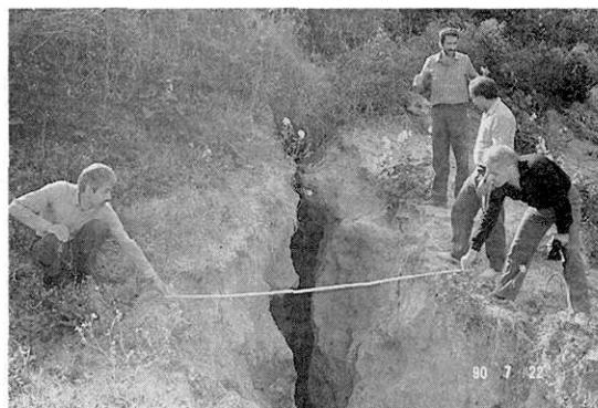
Photo 29. The largest open crack on the second terrace of grassland in Pakdeh (Site No. 2 in Fig. 8). Looking west.
