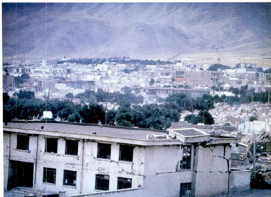
Photo 5. Close-up view of the City of Manjil. Almost all the buildings were destroyed completely or beyond repair. The scene looked as if a giant had crushed them under his foot.
