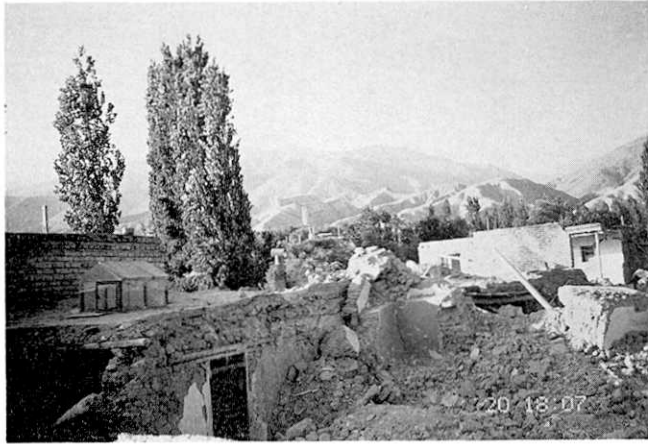
Photo 6. Ganbarabad area in the town of Abbar. Looking north. Mud-brick houses collapsed. A two-storied burned-brick house with a wooden frame at the back stood, suffering relatively light damage. 45 people were killed among the total 400 population in this area.
