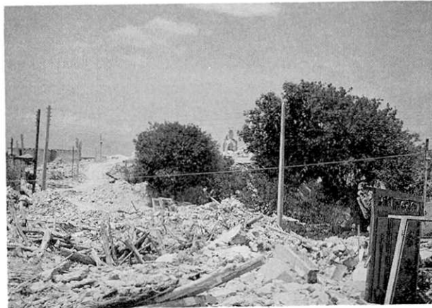
Photo 7. Bivarzin Village on the spur of a hill. Looking south. The loss of lives amounted to 47% of the 638 inhabitants. On the top of the hill is a destroyed mosque as shown in Photo 8. Utility poles remained undamaged.
