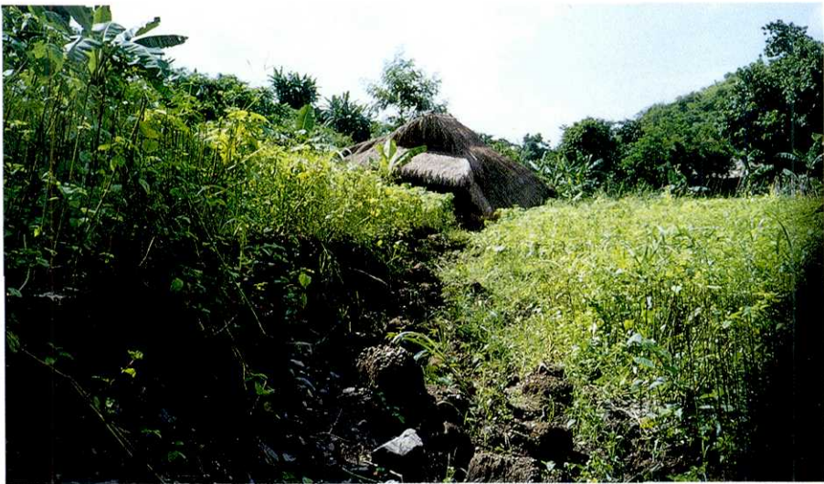
Photo 6. View looking southeast along exposed fault south of Puncan. Horizontal and vertical displacements are 5 m and 1 m. The ground was horizontally tensiled by 1 m across the fault. A nipa house on the fault was scissored.
