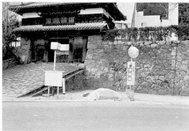
Fig. 13. The 1707 Nankaido tsunami inundated 2.7~3.0 m (above ground) under the gate of Saiki Castle and 4 persons were drowned in the town.
