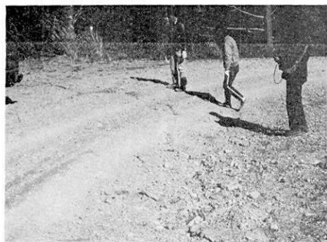
Fig. 30. En echelon cracks at Loc. b (1 km northeast of Takigoshi).
