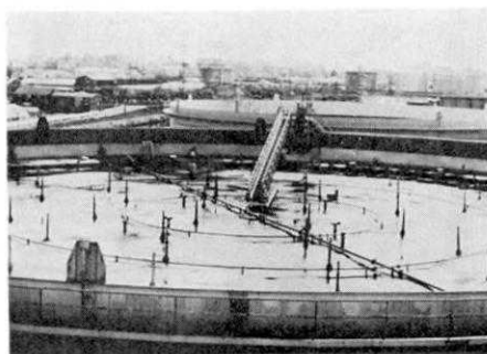
Photo. 7. Damage of rolling ladder on the roof.
