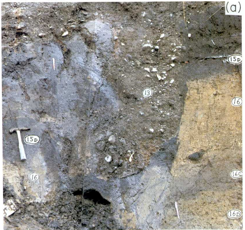
Fig. 31. Pocket filled with gravel in the main fault zone [AN 6~7-7~10]. The location is shown in attached sketch, (a).
