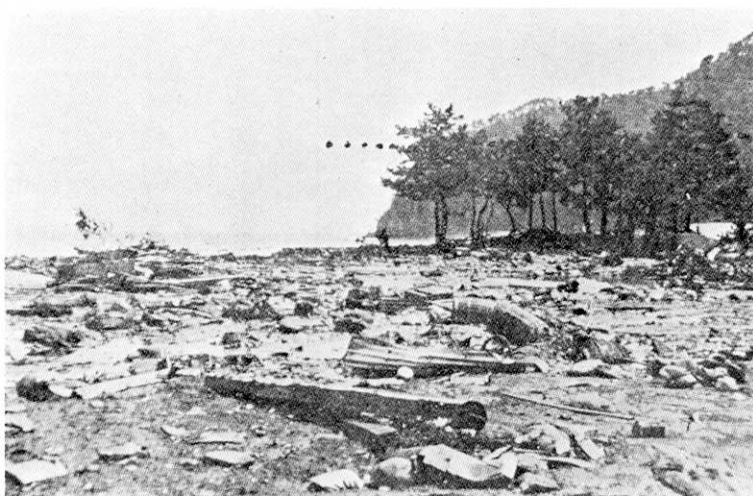
Fig. 2. Damage to houses caused by the 1923 Kanto tsunami at Atami (from T. Ikeda). The dotted line shows the inundation level (12.0 m above sea level).
