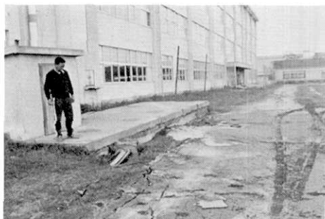
Fig. 24. Buoyed septic tank beside the school building (Noshiro Shogyo High School).
