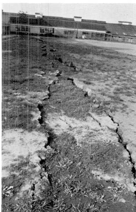
Fig. 25. Ground Cracks (Noshiro Shogyo High School).
