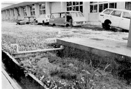
Fig. 19. Buoyed septic tank due to liquefaction (Oga Kogyo High School).
