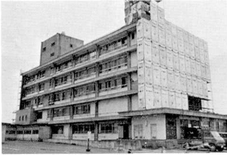
Fig. 2. North elevation of Namioka town hospital (Namioka-cho, Aomori pref.).
