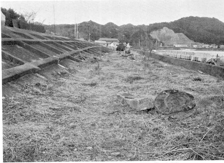
Fig. 9. General view of the sea wall at Hiro.
