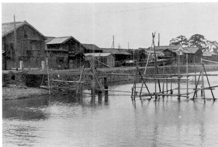
Fig. 3. Bridge destroyed by the 1946 Nankaido tsunami near the mouth of Yamada River, Yuasa (Photo taken by R. Takahasi).
