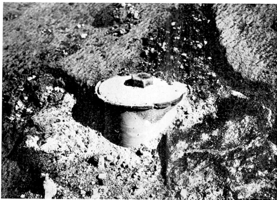
Fig. 13. A part of the polyvinyl chloride pipe of a bench mark on the summit was melted.
