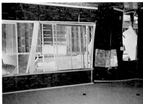
Fig. 28. Inside of the drive-in restaurant.
