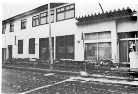
Fig. 24. Collapsed block fence. (photographed by Urakawa town office.)
