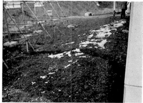
Fig. 53. Crack on ground in Mitsubishi town.
