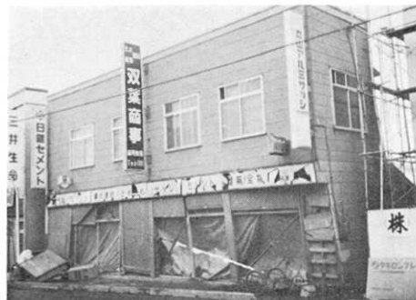
Fig. 13. Damage to a shop in Tokiwamachi.
