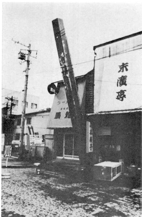
Fig. 23. Leaning chimney. (photographed by Urakawa town office.)
