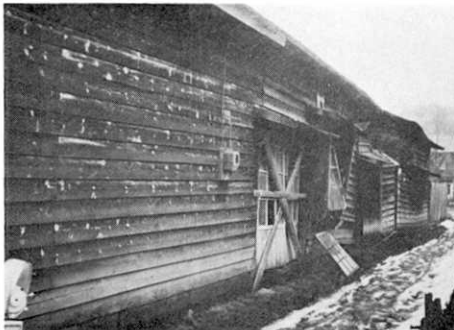
Fig. 12. Damage to old wooden house in Tokiwachi.
