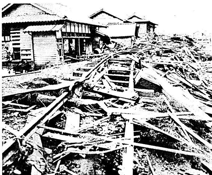
Fig. 3b. Damage of the railway caused by the 1960 Chile tsunami at Dai-machi, Ofunato (courtesy of Asahi Press).
