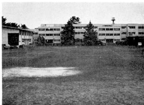
Fig. 2. North elevation of Futo Elementary School Building and Gymnasium.
