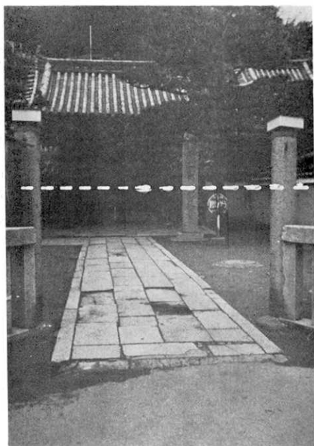
Fig. 7a. Inundation level (broken line) of the 1854 Ansei tsunami at the Eishoji Temple in Kainan. Tsunami height is 4 m above M. S. L.
