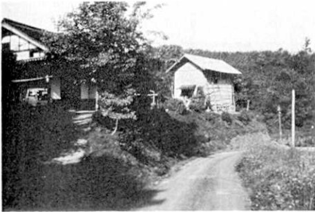
Fig. 24. Small mud-wooden warehouse on the narrow embankment was damaged. This damage seems to be affected by the lay of the site.
