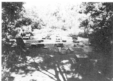
Fig. 20. Fallen grave stones to the almost same direction in the cemetery located on top of a narrow hill about 10 m high. (Sensho Temple graveyard, Sanbe hot spring). This fact shows topographical effects on the intensity of ground motion.
