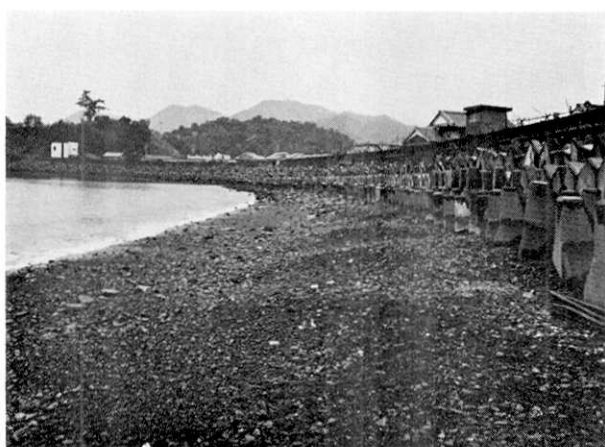
Fig. 10a. General view of the sea wall which surrounds Nieura town. Inundation heights were as follows; the 1707 Hōei tsunami: 7–8 m, the 1854 Ansei tsunami: 6 m, and the 1944 Tonankai tsunami: 5 m.
