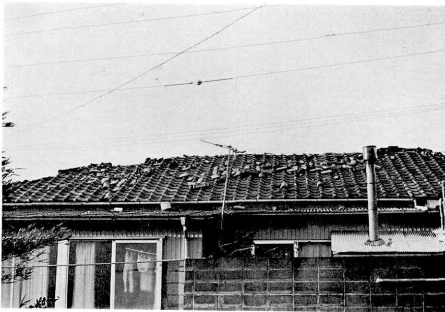
Fig. 13. Damage to a tiled roof at Moto-machi, Oshima.
