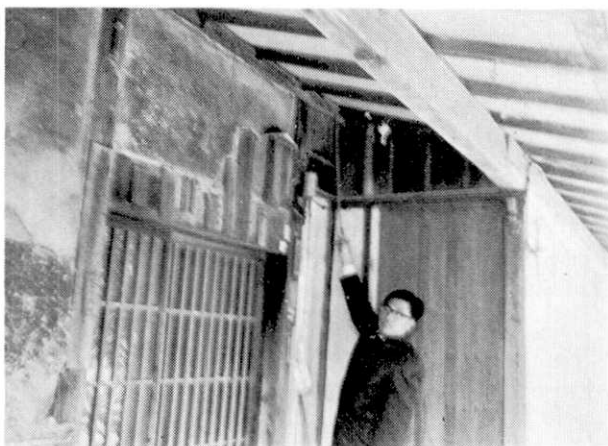
Fig. 11b. Trace of the inundation level (7.2 m above M.S.L.) of the 1854 Ansei tsunami at Tabi.
