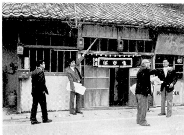
Fig. 17b. Trace of the inundation level (5.6 m above M.S.L.) of the 1854 Ansei tsunami at Maisaka.
