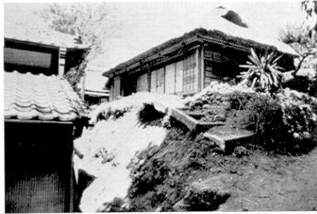
Fig. 11. House damaged by collapse of a slope.
