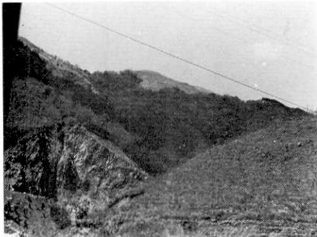
Fig. 59 a. Damagl at Hata, fissures in the rock and in the ground.
