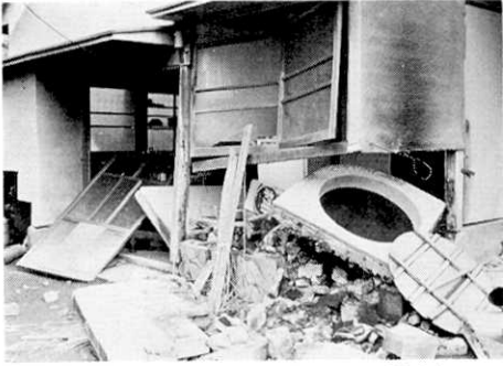
Fig. 47. Damage to a house at Uchiyama (Mrs. Chiyoko Kawano's house).
