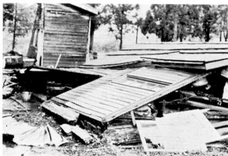
Fig. 13. Collapse of a warehouse of a school at Teradoko.
