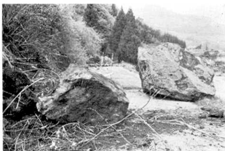
Fig. 33. Fallen stones on a road at Tabuse.
