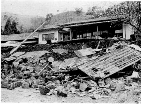
Fig. 42. Destruction of stone wall at Uchiyama.
