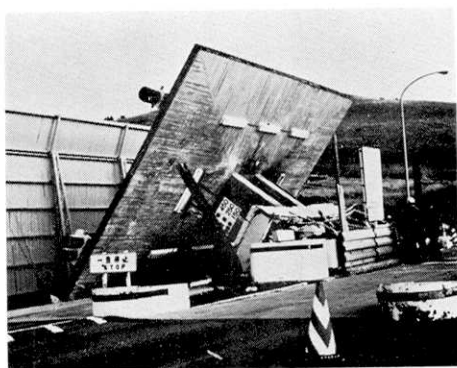
Fig. 18. Collapse of a toll-gate of the Yamanami Highway at the side of Yamashita-ike.
