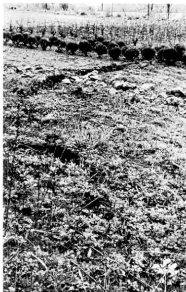
Fig. 15. Fissures in the ground at Teradoko.
