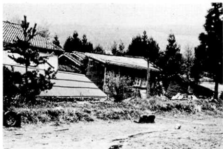
Fig. 12. Destruction of a school at Teradoko.
