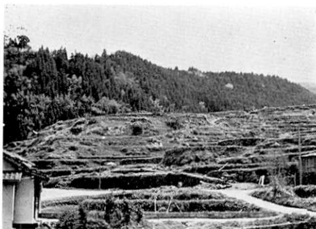
Fig. 32. Sliding of the supporting soil of rice-fields at Kagono.
