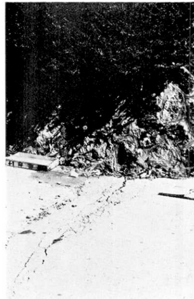
Fig. 26. Fissures in the ground by Lakeside Hotel at the side of Yamashita-ike.
