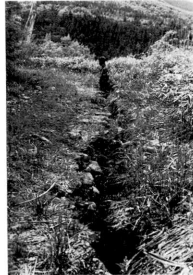
Fig. 41. A fissure on a road near Ogiyama.
