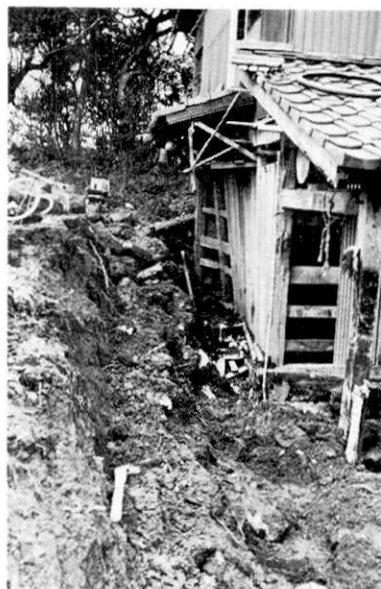
Fig. 55. Sliding of loose pyroclastic sediment at Shiode.
