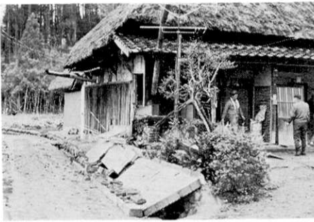
Fig. 8. Destruction of a block fence at Okunameshi.
