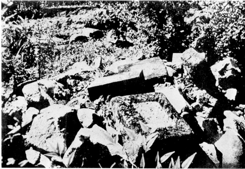
Fig. 11. Example of gravestones fallen down. (Hatasa section, Okumyogata)
