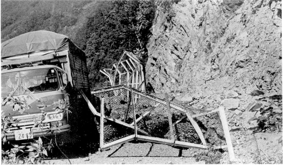
Fig. 10. The stone fell down on a truck. (Route 156, the national road, Aioi sections, Gujyohachiman)
