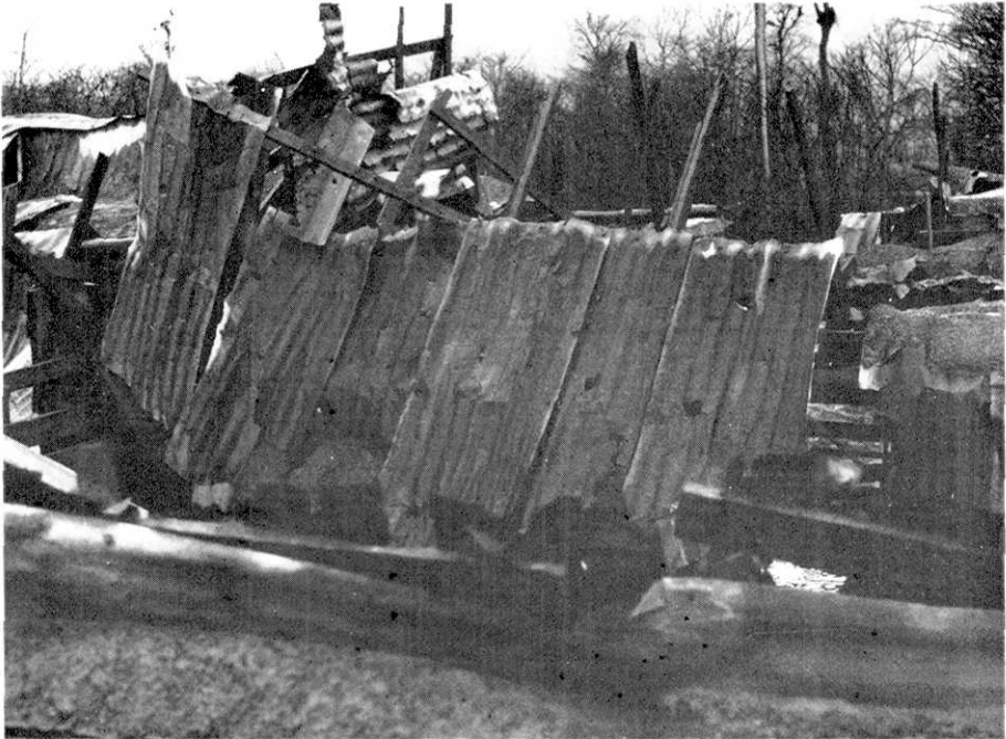
Fig. 21. The houses and cottages destroyed by the fall of the abundant fine ejecta of July 29 at Pueblo Nuevo.
