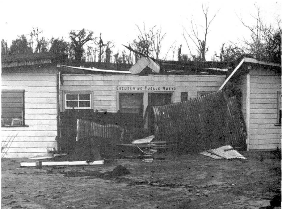
Fig. 22. The houses and cottages destroyed by the fall of the abundant fine ejecta of July 29 at Pueblo Nuevo.
