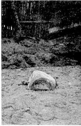
Fig. 2. An example of damaged bench mark.
