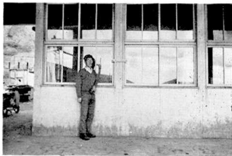
Fig. 7. The level of the maximum wave at the office of a fisheries cooperative in Kuji.
