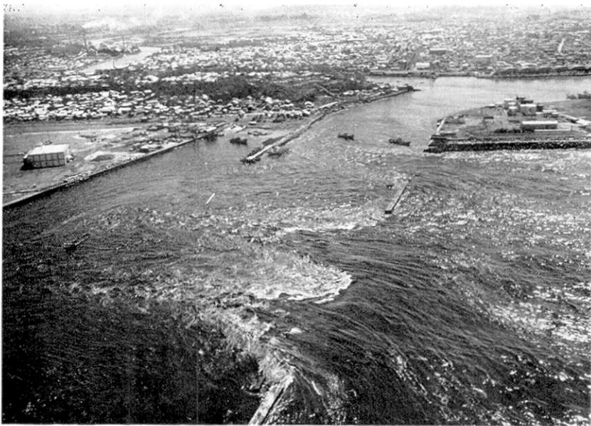
Fig. 5. Tsunami flowing into Hachinohe Harbor through a gap in the damaged breakwater (courtesy of Yomiuri Press).
